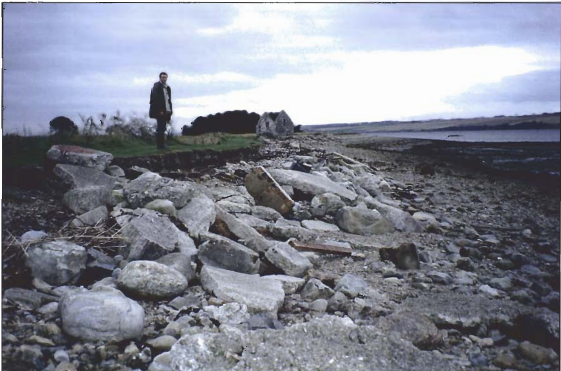
Plate 2. Kilmuir foreshore showing dump defence and erosion.
