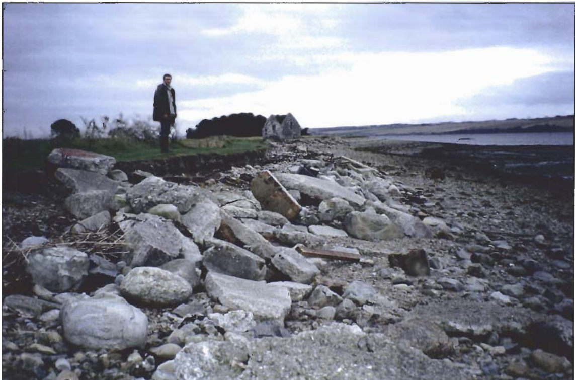
Plate 2. Kilmuir foreshore showing dump defence and erosion.
