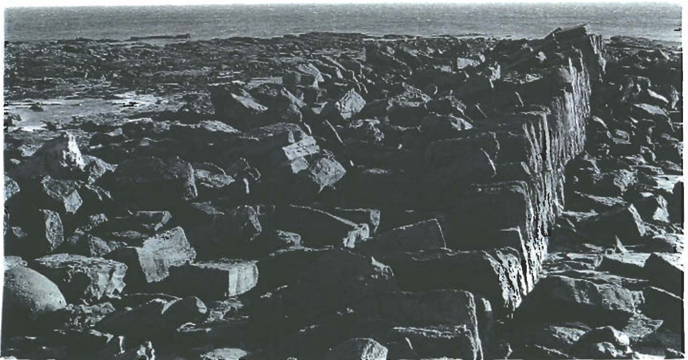
Fig 6: Kingsbarns harbour wall looking east Photograph - Rudiger Bahr
