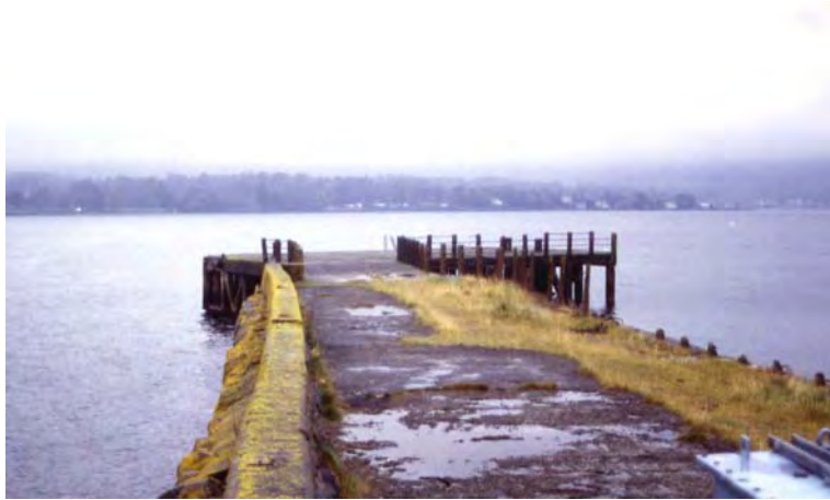
Plate 3: Site C41: Strone Pier.
