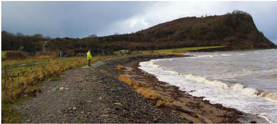
Plate 13: Defensive gravel ramp and erosional face to north of the Heads of Ayr.
