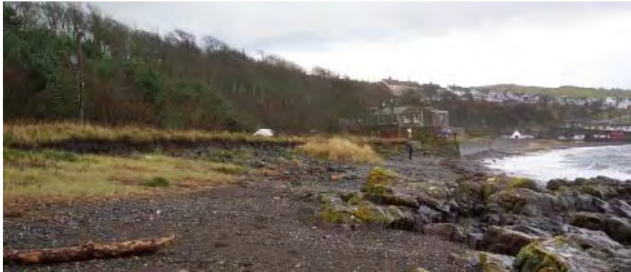
Plate 12: Erosional nick to north of sea wall at Dunure.
