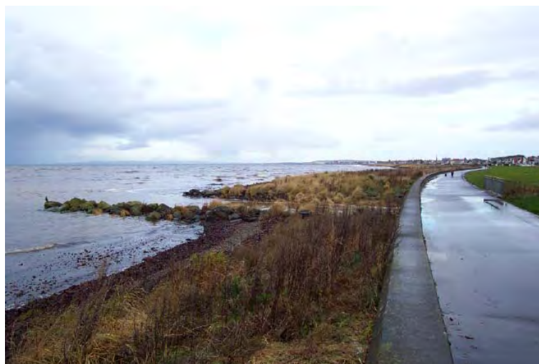
Plate 14: Slaphouse burn lined with geotextiles and riprap groynes.
